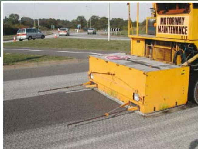
(Above) Retexturing processes are generally not plant and process-intensive, producing a smaller carbon footprint. Traffic management is less onerous and there is less disruption to motorists.
