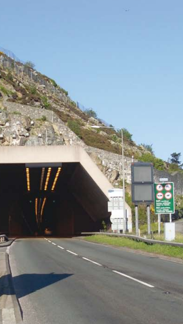
As well as restoring skid-resistance, bush hammering has been found effective in removing hydrocarbon deposits from road sections through tunnels. Photo shows the Pen-Y-Clip tunnel on the A55 in North Wales. Photo courtesy of North Wales Trunk Road Agency.
